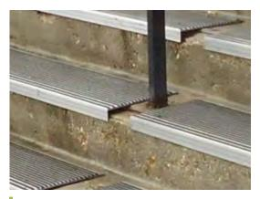
Photo 78: Loose exterior stair treads
