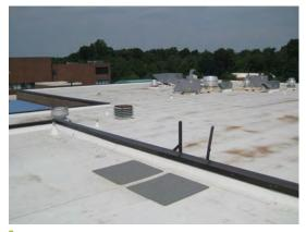
Photo 19: TPO Roof and Access Ladder
