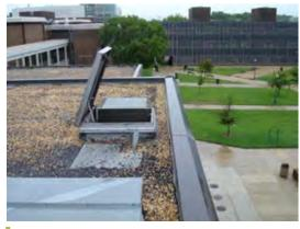
Photo 75: Serious fall hazard at roof hatch
