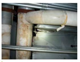
Photo 56: Damaged ductwork on AHU-2
