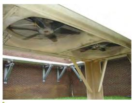
Photo 58: Safety hazard on cooling tower. Fan guards are removed with fans running.
