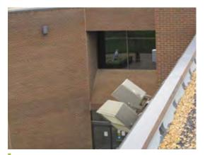
Photo 13: Lights surfaced-mounted on exterior walls
