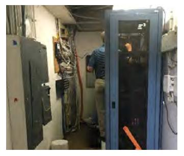
The entire building is served by a telecommunications room on the Second Floor. The room is long and narrow, not the ideal size and shape for today's telecommunications rooms. Due to a lack of storage in the building, both the entrance location and the telecommunications room have a lot of clutter, with boxes, chairs, HVAC filters, etc. blocking easy access and passage. Backbone and horizontal cables supporting data, voice, and video services route from their device locations to this room.
