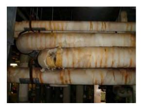
Photo 53: Damaged chilled water pipe insulation
