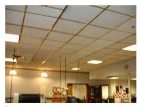
Photo 76: T-12 lights should be replaced by T-8s
