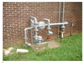
Photo 63: Natural gas meter and regulator
