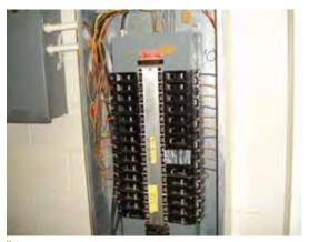
Photo 66: Pacific Electric panel with missing front shield & exposed wiring in room 241
